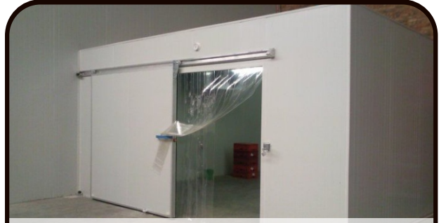
Cold Storage Room
